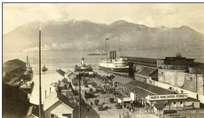
SS Prince Albert – North and West Vancouver Ferry Docks
